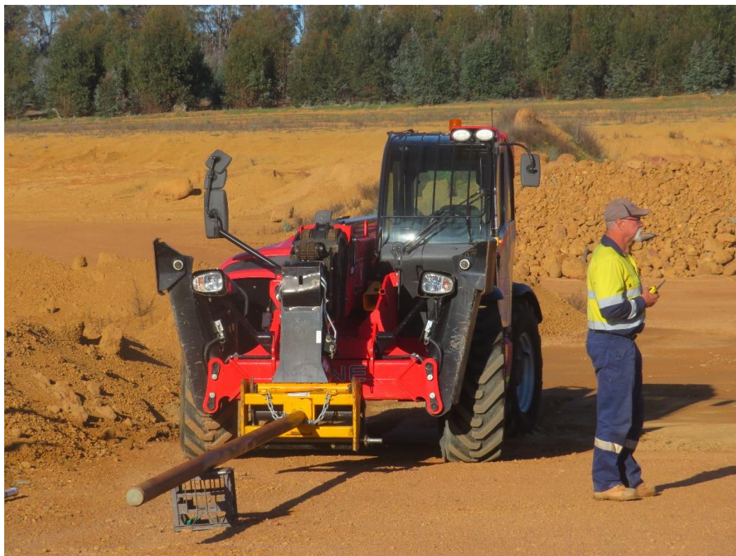
Figure 9. Manitou 1840 telehandler fitted with steel-prong used to install monitoring tubes into the gravel stockpiles during the trial.
