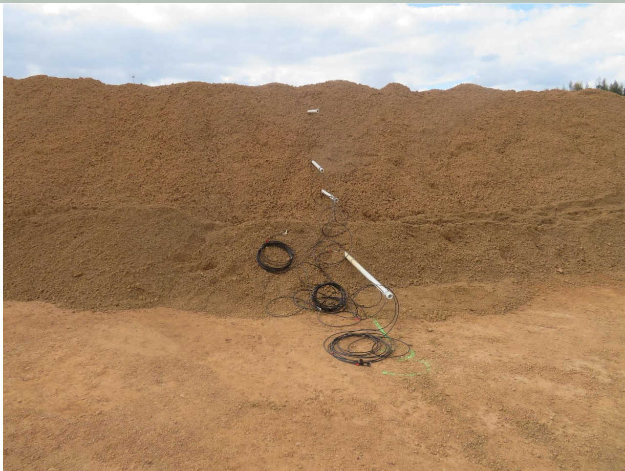
Figure 6. Intergranular MITC monitoring probes installed within the treated stockpile. Sampling lines were inserted through the slotted PVC tube infrastructure at predefined heights and lateral distances (Figure 7, Figure 8), with surface tubing connected to field gas-monitoring equipment for measurement of methyl isothiocyanate (MITC) concentrations within the gravel matrix.
