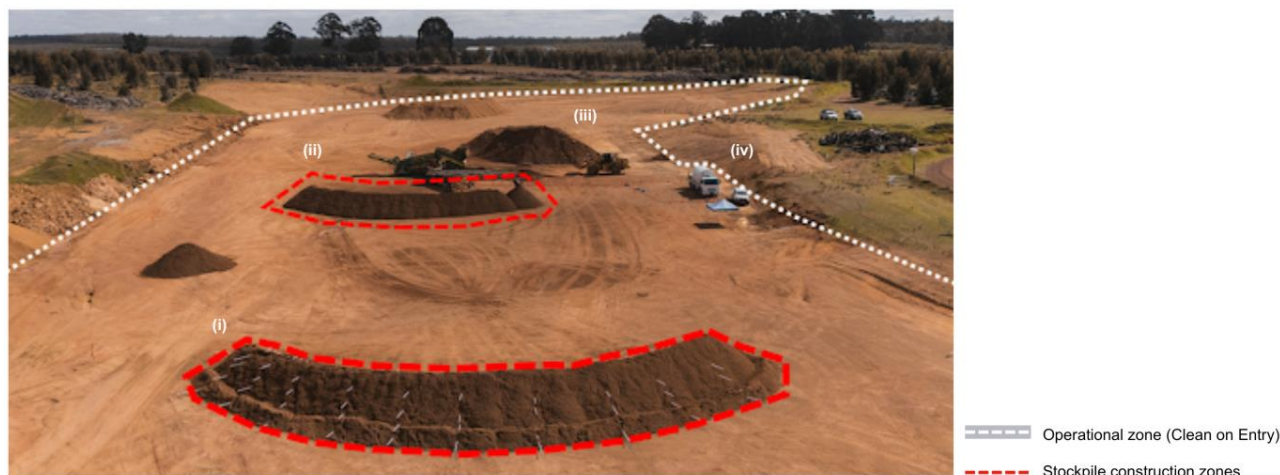
Figure 3. Drone image depicting site layout at the Culford Agri Industry Precinct, North Bannister, WA. The dotted white line delineates the operational zone, within which all access was strictly managed for dieback hygiene. Within the operational boundary, the control stockpile (i), treated stockpile (ii), source material (iii), and chemical treatment truck (iv) can be observed. The treated and control stockpile construction zones are demarcated by a red dashed line and were managed in accordance with uninfested pit management protocols (DBCA, 2020).
